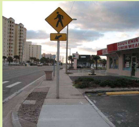
A sign pole is located within the sidewalk on SR A1A
