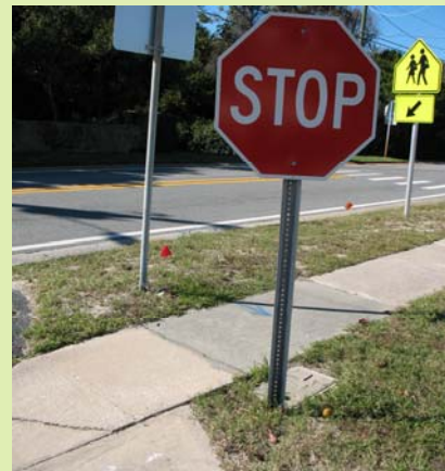
The stop sign at the exit onto Peninsula Drive is mounted too low
