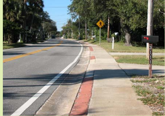
Red markings differentiate the roadway from the sidewalk along some sections of Peninsula Drive
